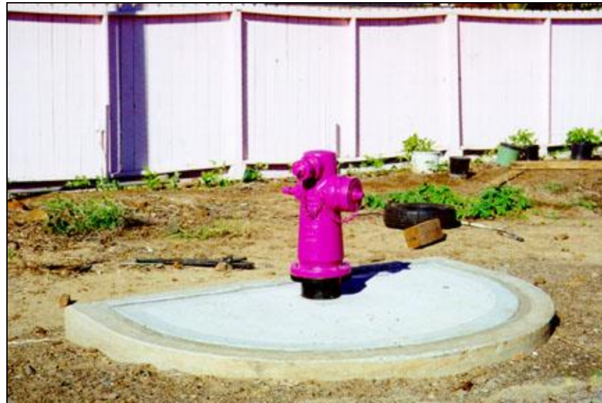
Reclaimed water hydrant (purple pipes)
