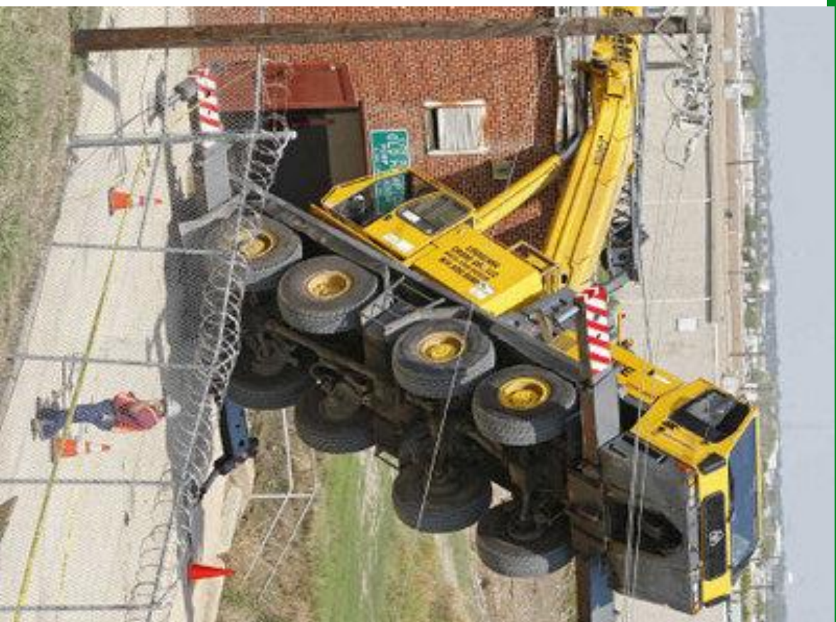
Maintenance: Rigging and Lifting
