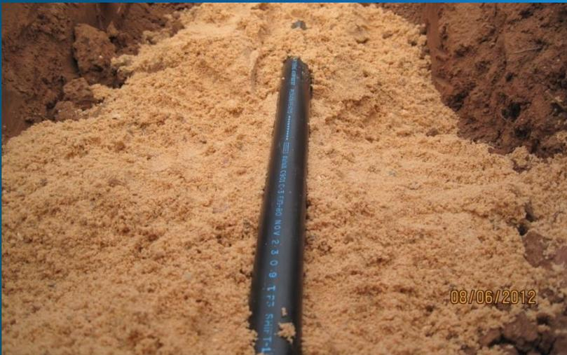
HDPE pipe requires sand backfill in rocky soils
