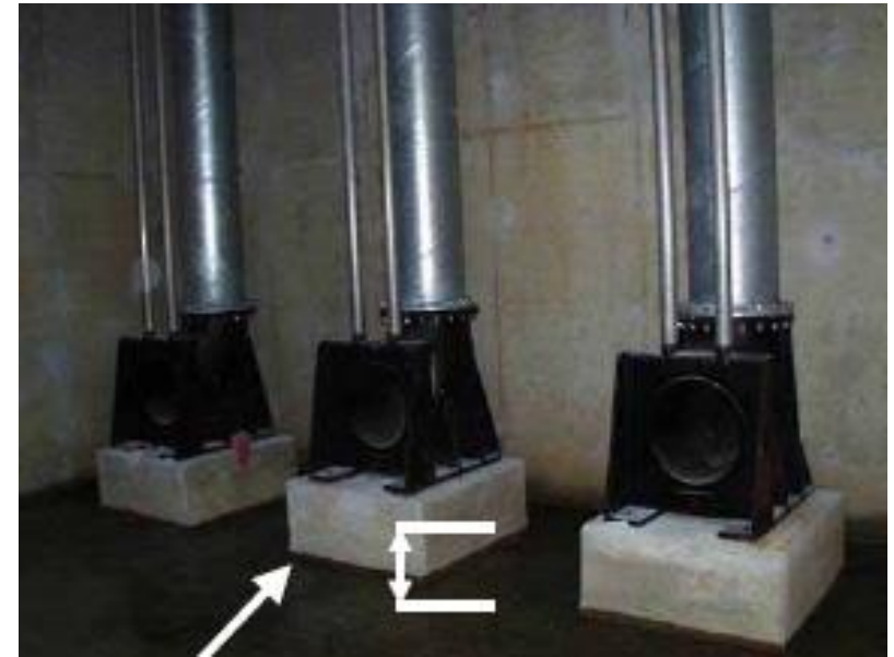
Proper pump arrangement
