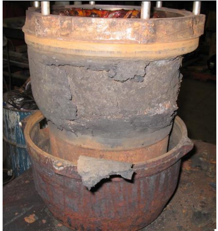
Open loop cooling system
