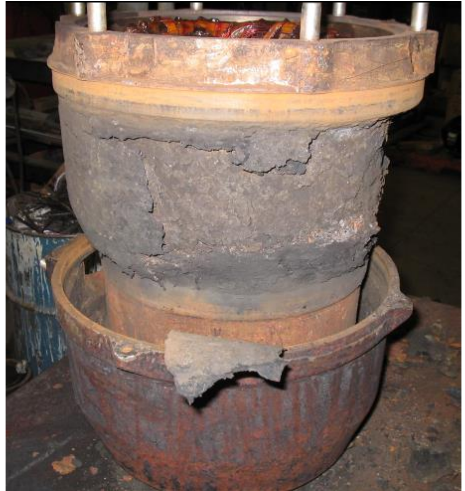
Open loop cooling system
