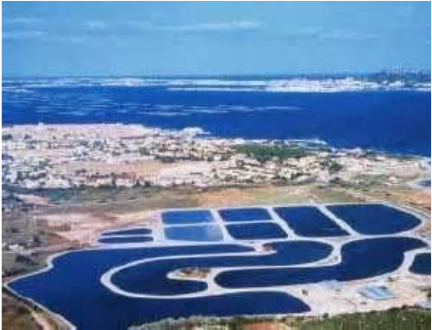
Waste Stabilization Pond
