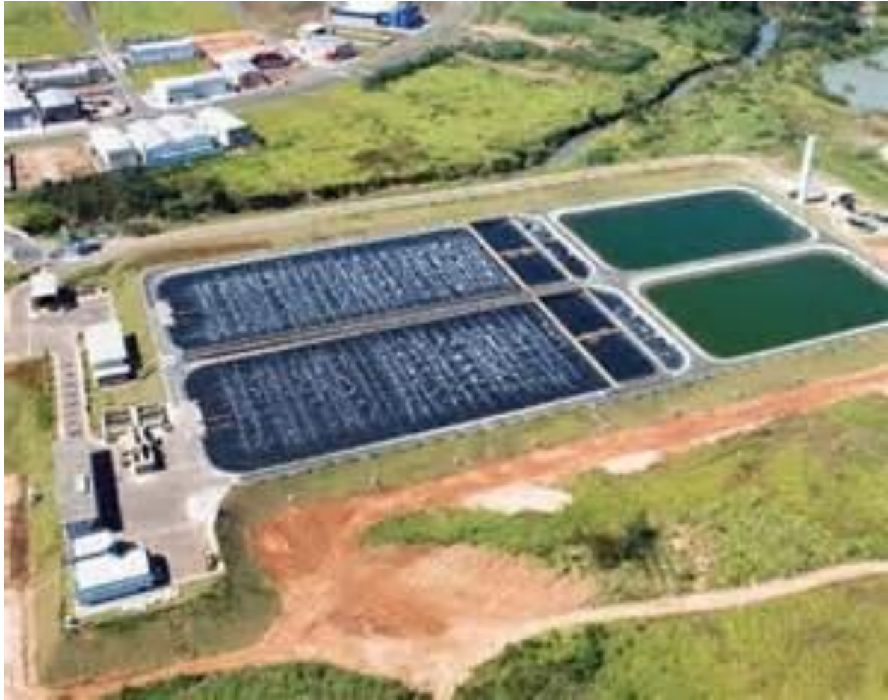
Extended Aeration Plant
