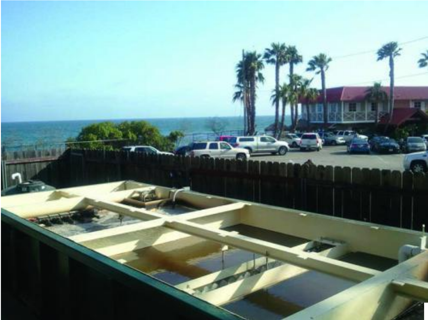
Malibu Restaurant-Onsite installer
