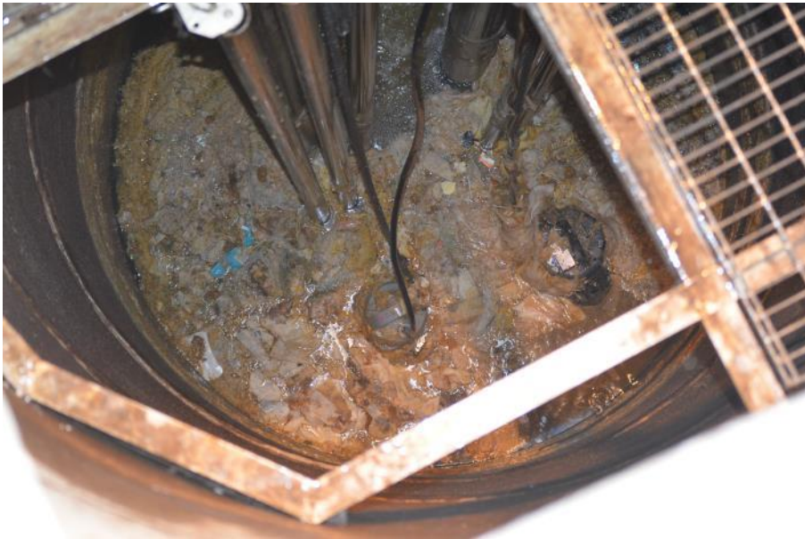
Before installing Concertor
