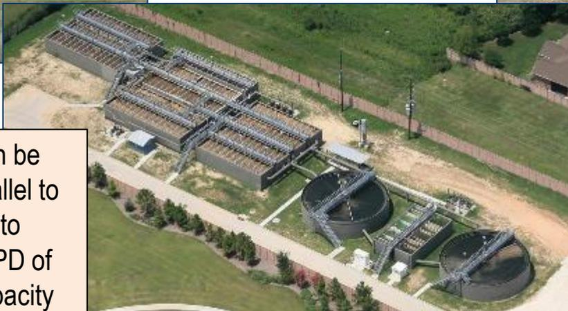
Modules can be placed in parallel to deliver up to 1,500,000 GPD of treatment capacity
