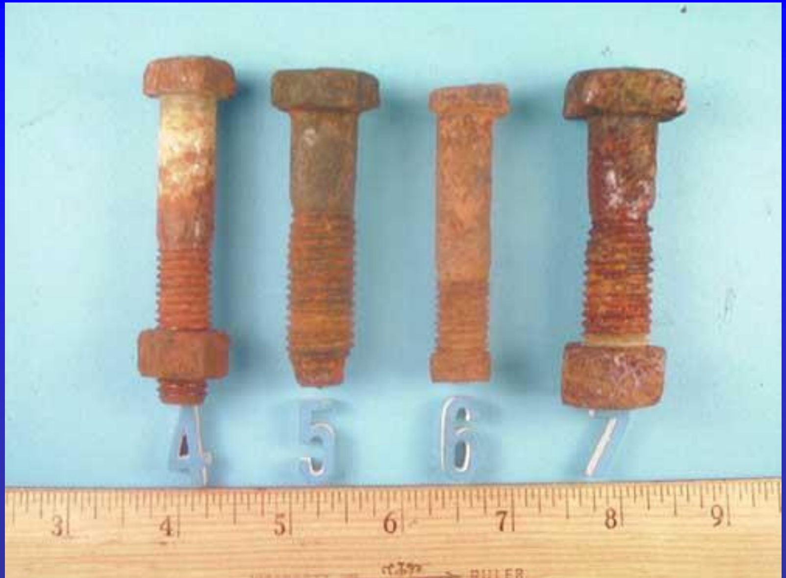
Bolt & Nut Corrosion
