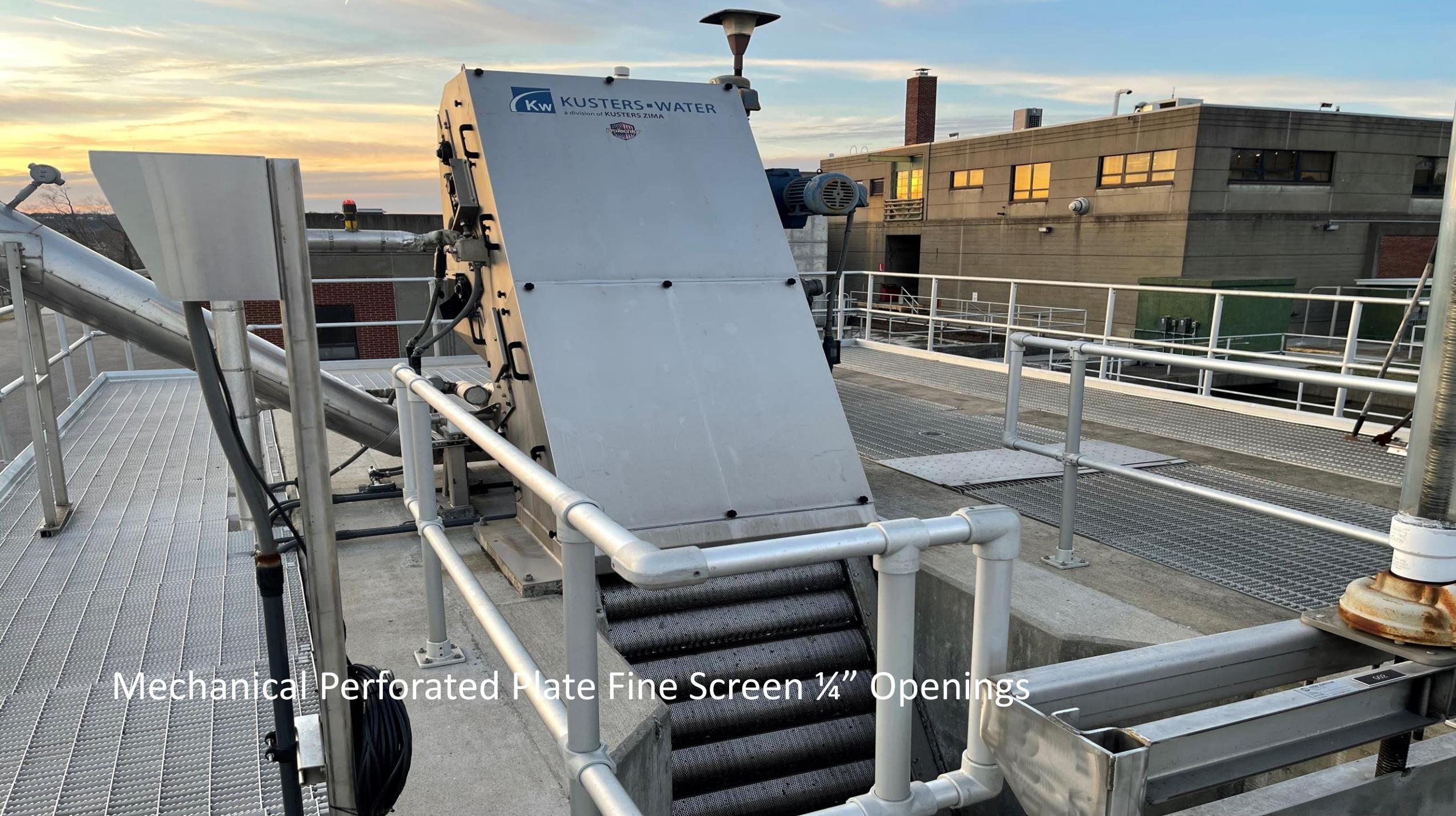
Mechanical Perforated Plate Fine Screen  $\frac{1}{4}$ " Openings
