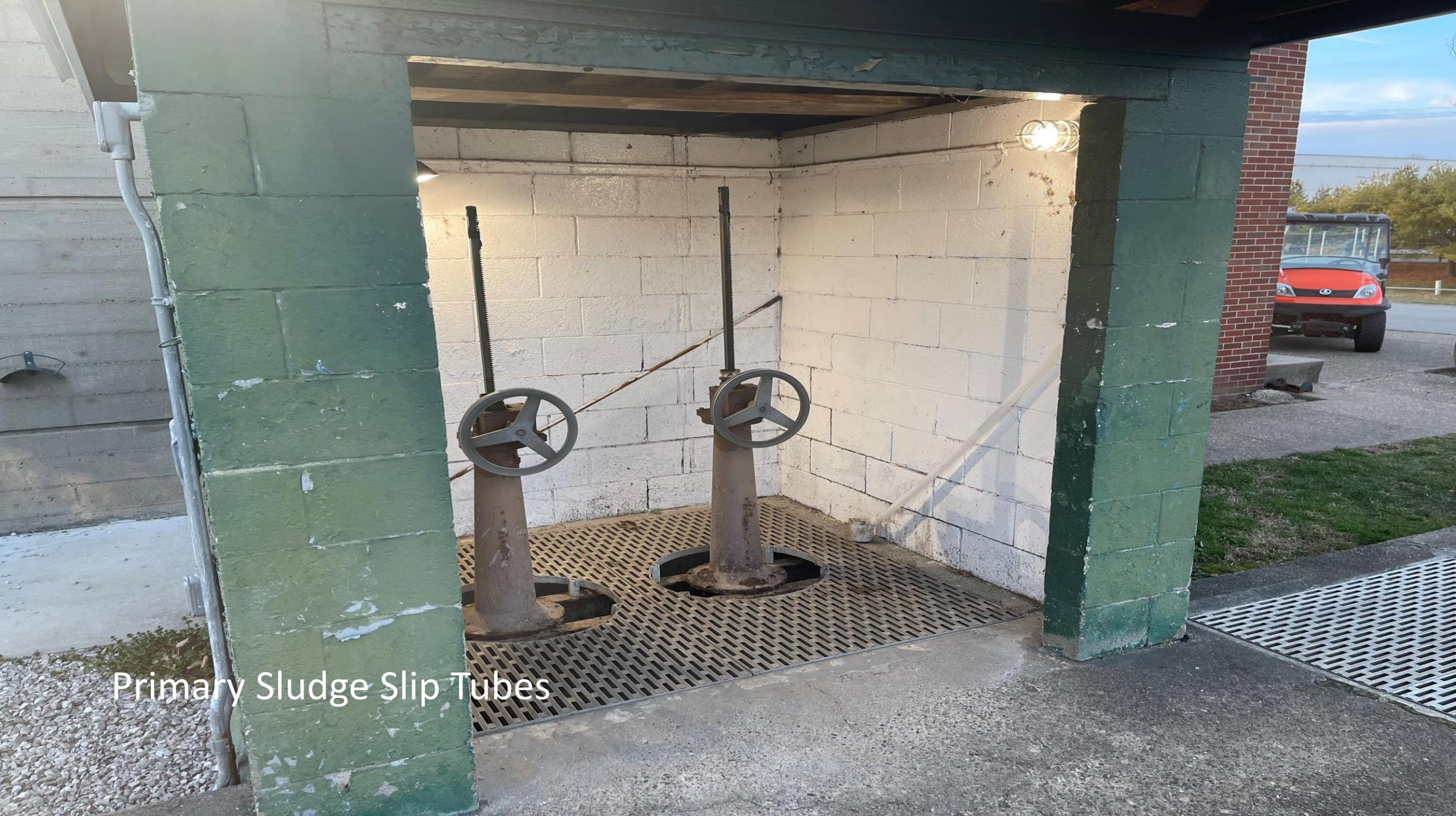
The image shows two manual slip tubes for primary sludge. Each unit consists of a vertical cast-iron shaft with a hand-cranked wheel at the top. The shafts are mounted on a metal grate floor. A thin metal rod connects the two wheels. The entire setup is housed in a small, enclosed space with light-colored cinder block walls and green-painted concrete pillars. A light fixture is mounted on the wall. In the background, a red utility vehicle is parked on a paved area.
