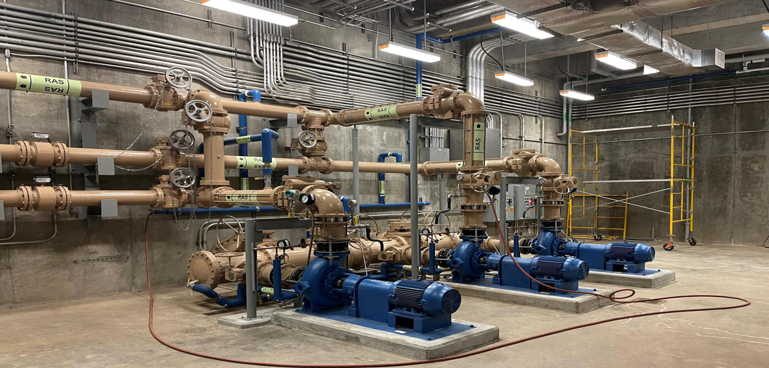
Hayward Gordon XCS Screw Centrifugal RAS Pumps (750-1500 gpm)
