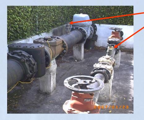
Test Taps for comparative testing
