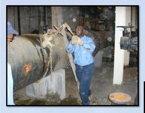
Pitot tap being installed inside the Plant
