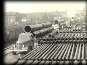
54" Diameter Iron Pipe Introduced (1965)
