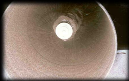
Cement Mortar Lining (1922)
