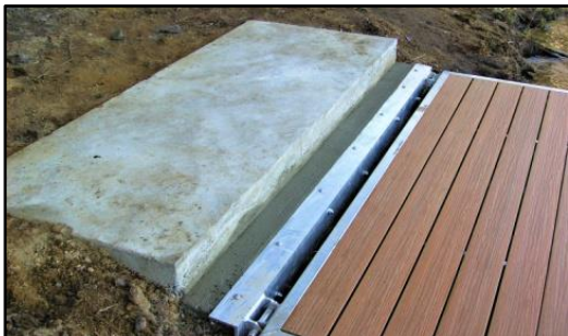
Concrete Angle on New Concrete
