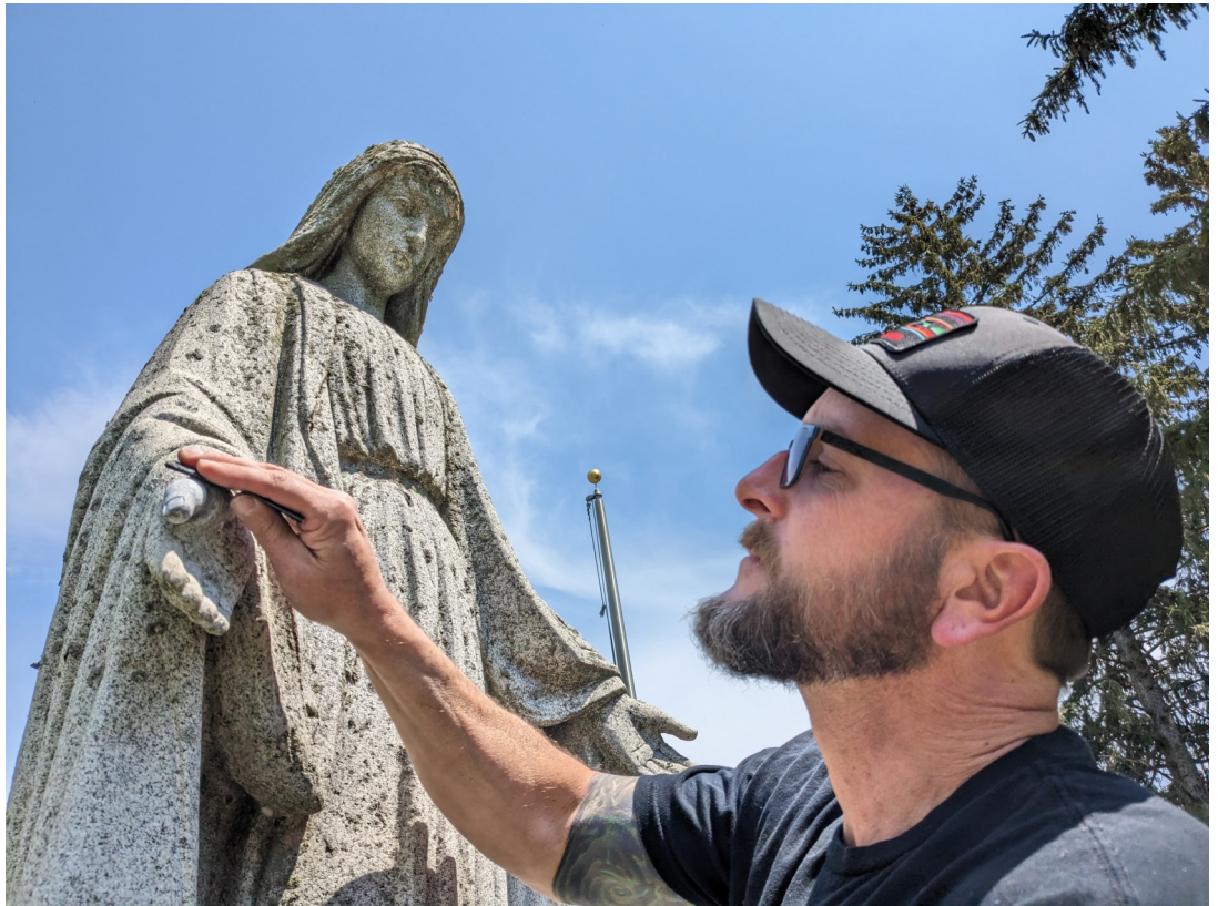
Dane Larsen does final polish on the thumb repair he performed on the monument to local veterans of the Blue Army at Holy Cross Cemetery.
