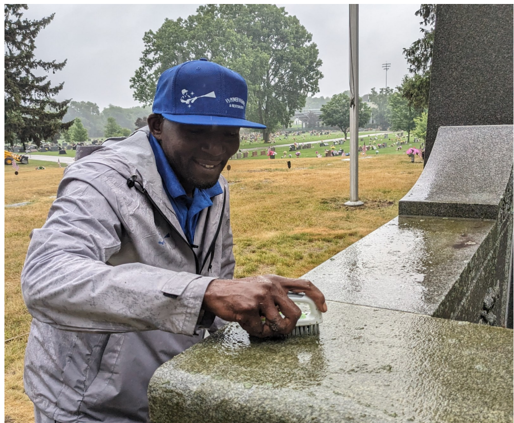
Sylvester Taylor uses a soft bristle brush and D/2 cleaner on base of the Polish army monument to remove lichens and mineral stains.
