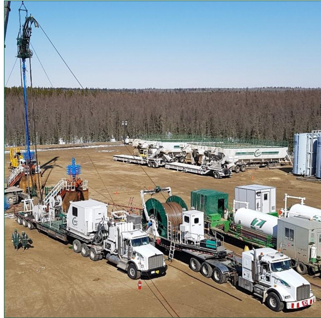
Coiled tubing operations in Canada. Calfrac Well Services Photos
