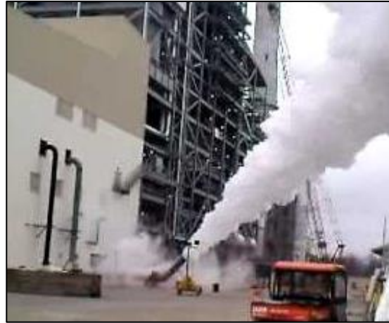
Noise from equipment & activities
