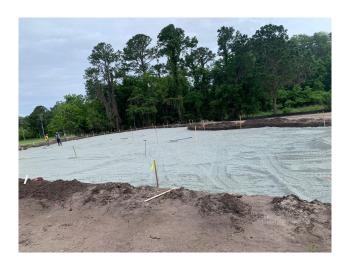
Grassing is on schedule for the middle of May. The Fairways will be sprigged with Tif Tuf, The greens will be sprigged with Tif Eagle, and the bunker faces will be sodded with Zorro Zoysia. The bottom of the bunkers are going to be at a 2-3% slope eliminating the flashing of sand faces. This has been an issue throughout the years and will speed recovery to playability after rain events.
