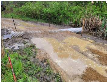
Work done on the East side of town replacing culvert. Thanks go out to Vertical Excavation for their help and all the volunteers!
