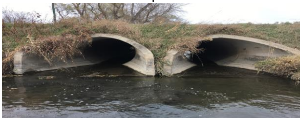
An example of one crossing in the historic channel that is undersized and set too high for water and sediment transport.
