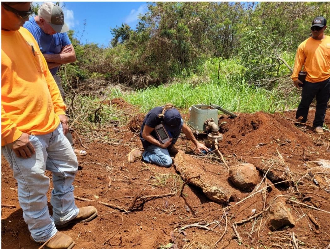
Placing the sensors on the steel pipes
