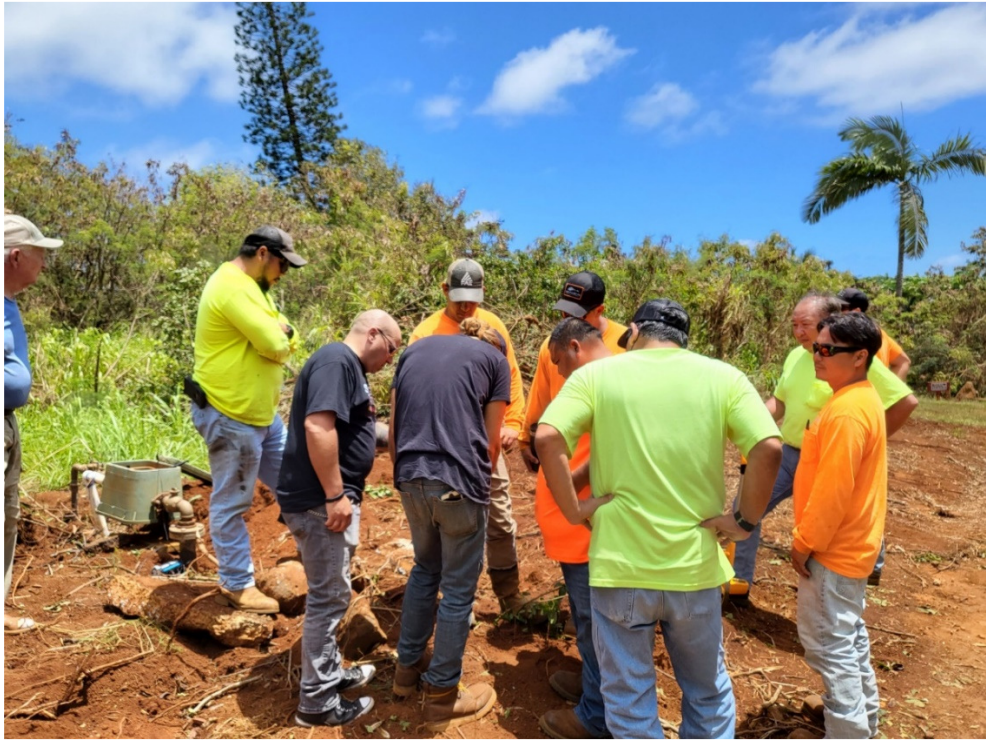
Hands-on with Leak Detection Training – Department of Water Field Crew in Orange/Green Shirts
