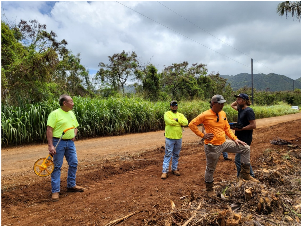
KDOW crew helping with measurements/pipe location
