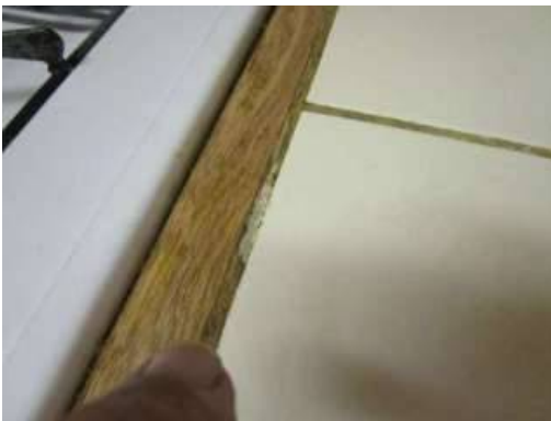
Photo 10-12 The grout needs to be repaired at the edge of the countertop.
