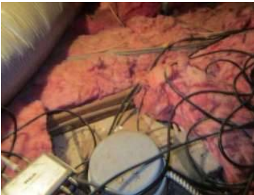
Photo 4-4 Many abandon tv cables have been left in the attic, you may want to remove. (this is not an issue).
