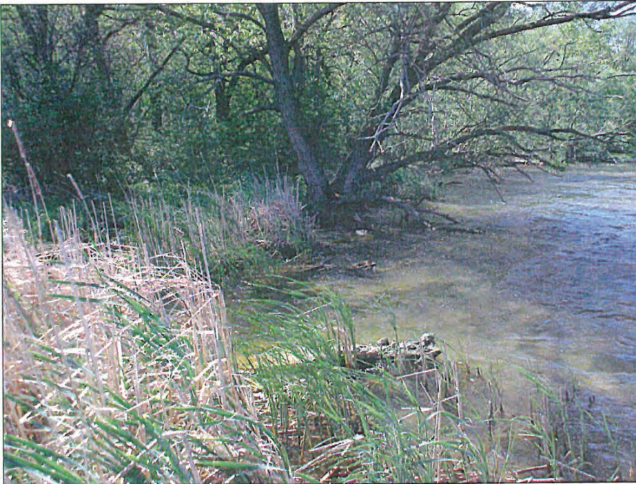
Photo #8 – Hooker Lake Dam (May 20, 2009)
