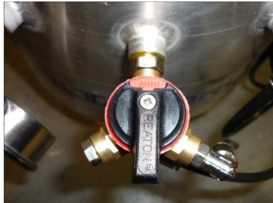
operating pressure of the system. Once the system is filled you will then be able to open the valve fully.
