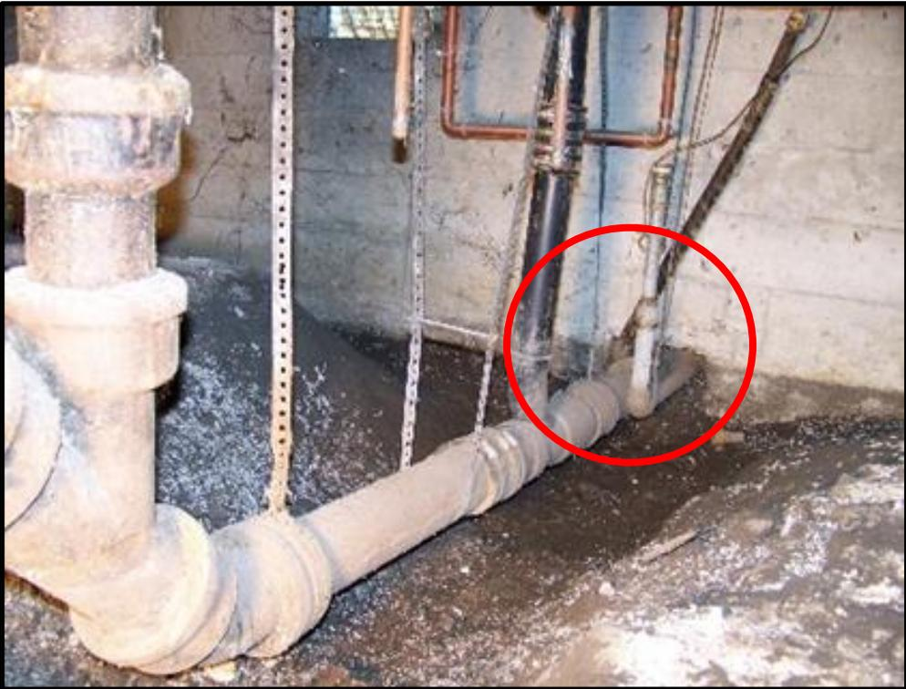
Current discharge of some sump pumps – pumps in almost all of the 163 buildings, all crawl spaces wet to varying degrees
