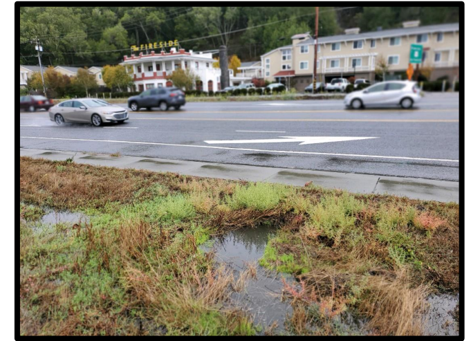
Ponded right of way, Manzanita
