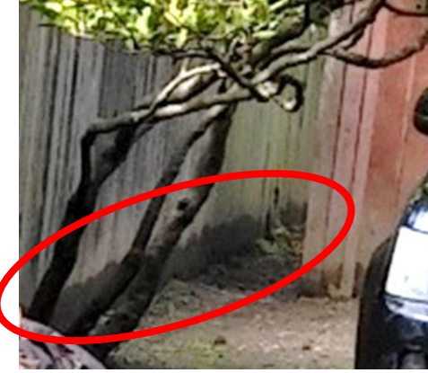
Water wicking up pavers, walls and fences
