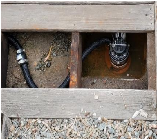
Sump pumps running constantly; discharge to the street (irrigation contribution?)
