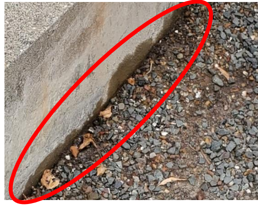
Water wicking up pavers, walls and fences
