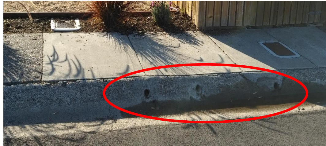
Sump pumps running constantly; discharge to the street (irrigation contribution?)
