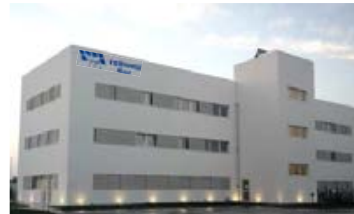
Tesmec Rail Monopoli-Bari Italy
