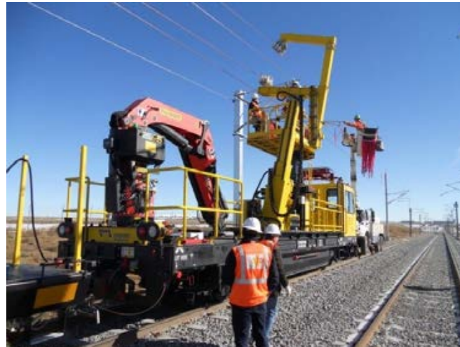
The wire train strings the overhead catenary wire on the East Rail Line, near 56th Avenue, in February 2014.
