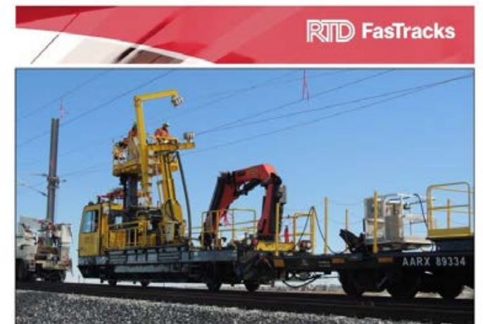
The wire train strings the overhead catenary wire on the East Rail Line, near 56th Avenue, in February 2014.
