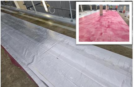
To the insulation, a VCL layer was applied which consists of an aluminium foil facer on top of a bitumen membrane – the Provap has a self adhesive backing.
