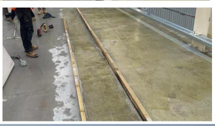
Three drainage channels were created, using insulation 40mm lower than the surrounding areas to reduce the chance of water pooling on the main roof, and to help aid the water filtereing into the channel. We used tannelised wood to create edge protection to prevent damage between the transition of 100mm and 60mm insulation.
