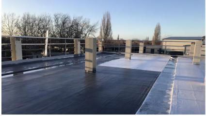
Once the PUMA membrane was installed, it is necessary to apply the 0.5kg/m2 EleRoof MME Top Coat FR to provide maximum fire performance and weather resistance.
