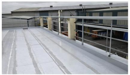
Due to the extreme weather – lots of rain, ice and strong winds during installation, the joints in the Provap VCL were feathered with PUMA Thixo as an effective night seal.
