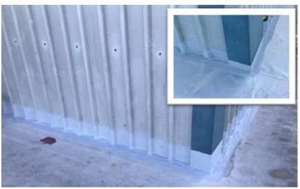
For the back edge connecting to the old building, it was important to waterproof to a high level. The gap was filled with rockwool to give linear gap fire performance vs PU foam or insulation. The rockwool was then coated with the PUMA Thixo membrane tanking up the wall.
