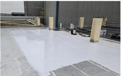
The next step was to start the installation of the 2mm PUMA elastic membrane with polyester fleece reinforcement. This provides the flexible layer in case of any movement.
