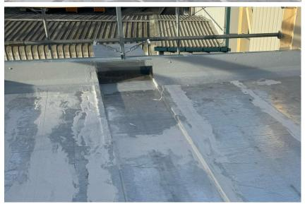
The façade goes up and over the metal perlins at the side and the client wanted a special detail around the perimeter – install a 200mm flexible GRP trim screwed to the metal (and later the cladding will be fixed through the top). The GRP was connected to the deck with a band of PUMA thixo under it and also 100mm fleece reinforcemed PUMA was applied to overlap the trim and the deck.
