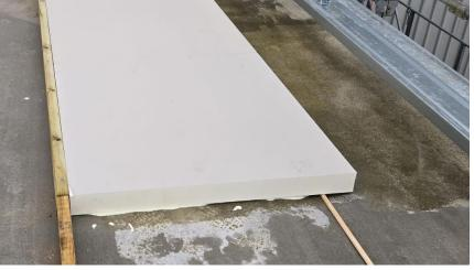
The insulation was started at the outer edge and we created a slight fall from the outer edge inwards to aid any flow of water in the future towards the drainage channels. We used PU foam adhesive to bond the insulation.
