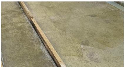
The next step was to apply EleRoof MMA Damp Prime to the surface, this works to seal in residual construction moisture from the concrete and providing a low MVT rate. The surface was aggregate blinded to enhance adhesion of the PU foam adhesive.
