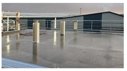
Commencing on the first week of January, the concrete literally had 5mm of pure ice over the whole deck. The first step was to start working on the edge detailing by melting the ice and flashing the concrete dry.
