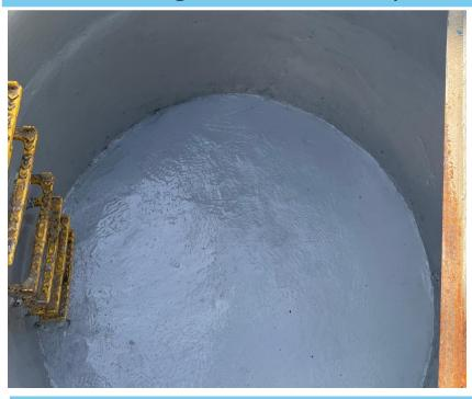
The large sump which held the rainwater, washing from the filling room, etc. was constantly exposed to diluted peroxide. Over time the surface wore away exposing large aggregates, slowly destroying the sump. We resurfaced the lining of the sump with Novolac Epoxy Mortar followed by 2 coats of Novolac Epoxy.
