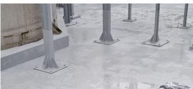
The peroxide bund was built in the case of accidental damage to the bunds that could result in a catastrophic failure and therefore fill the bund. The bund is a concrete structure.
