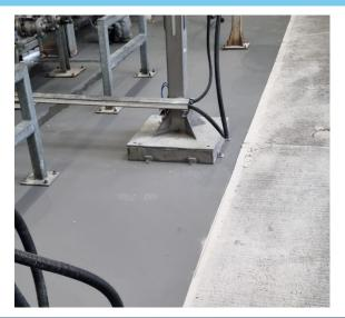
The filling room was used to fill drums from IBC containers. It is unavoidable to get drips and spills from time to time, and the floor was regularly washed down. Over time the concrete floor had started to be corroded.
