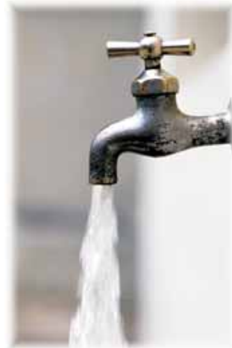
In the kitchen, check the water pressure, hot and cold water, and look for leaks.
