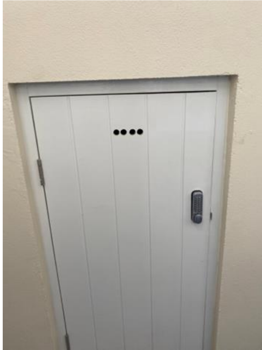
New Vault Lintels External [after]
