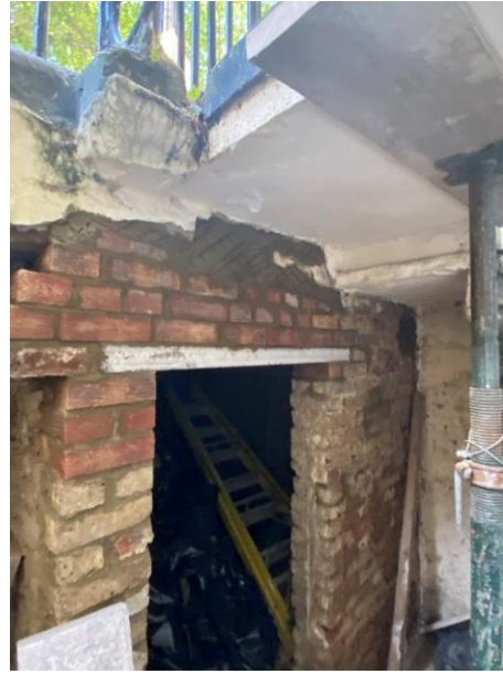
General Construction Photos
