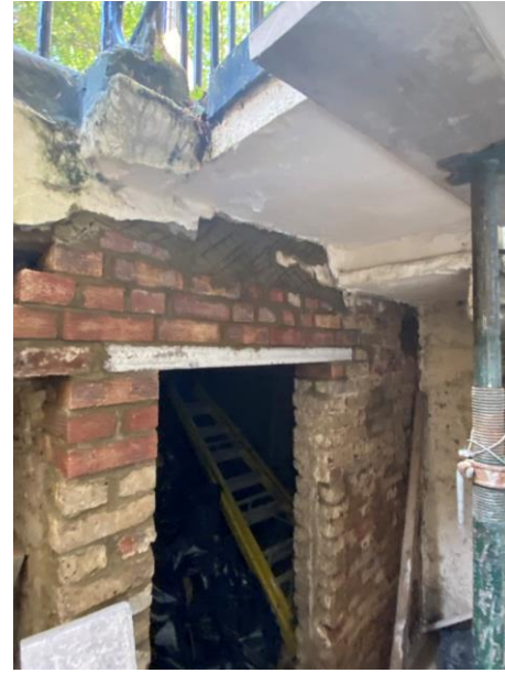
General Construction Photos
