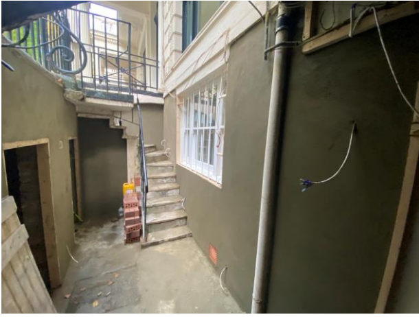
General Construction Photos
