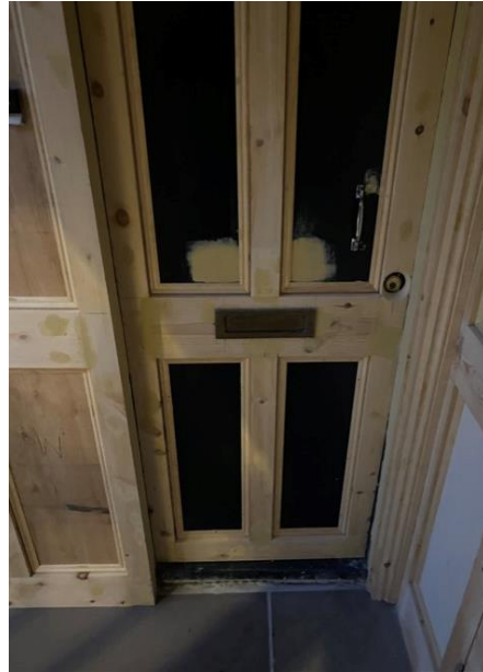
Existing LGF Entrance Reclad With Added Molding [during]
