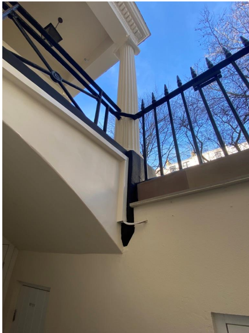
Structurally Underpinned Underside Portico [after]
