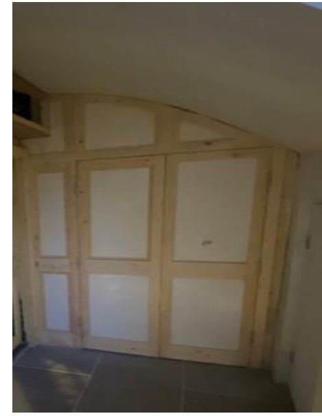
Existing LGF Gas Meter Cupboard Reclad With Added Molding [during]
