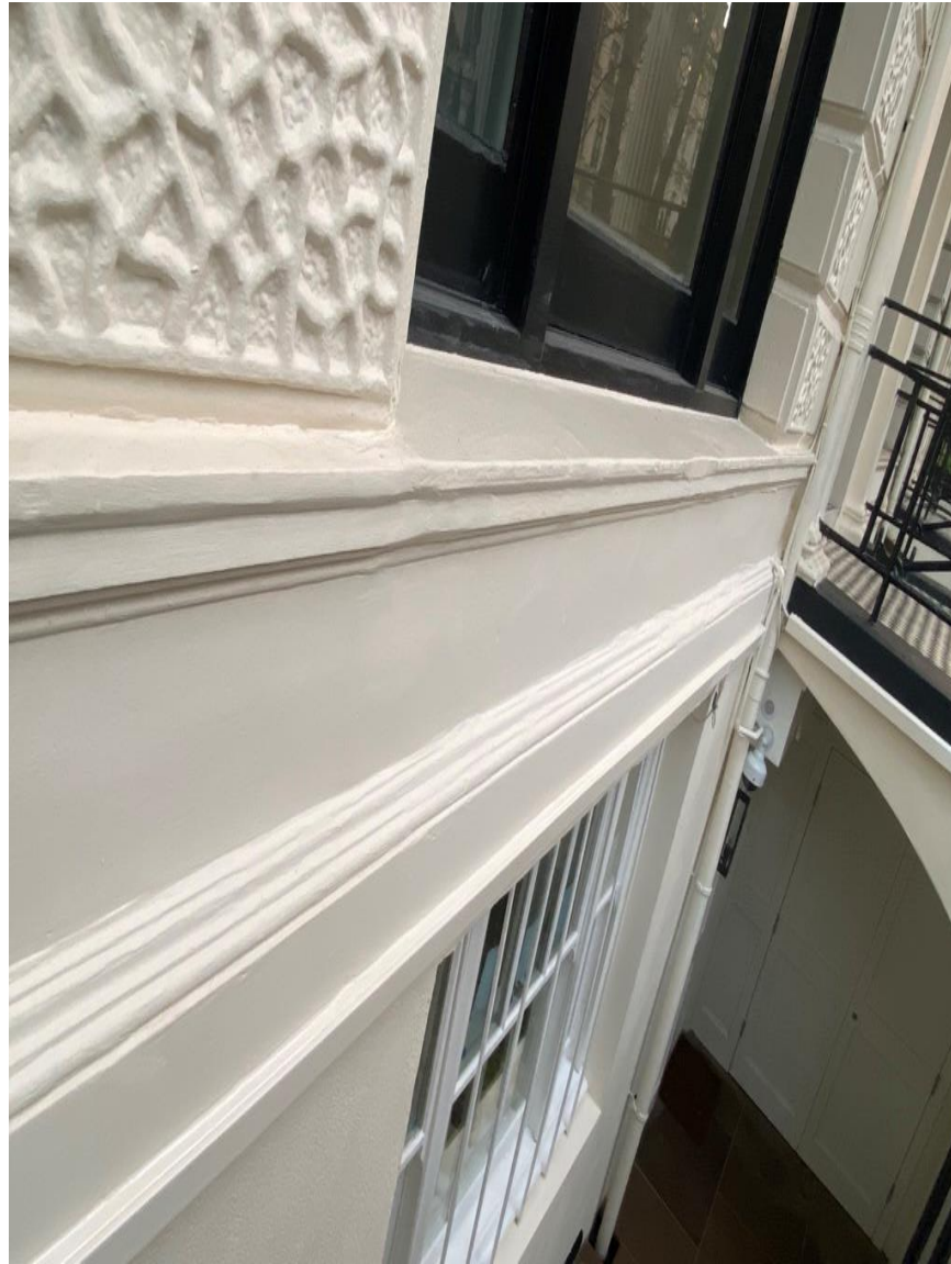
Restored Listed Sill Detail [after] including cable management
