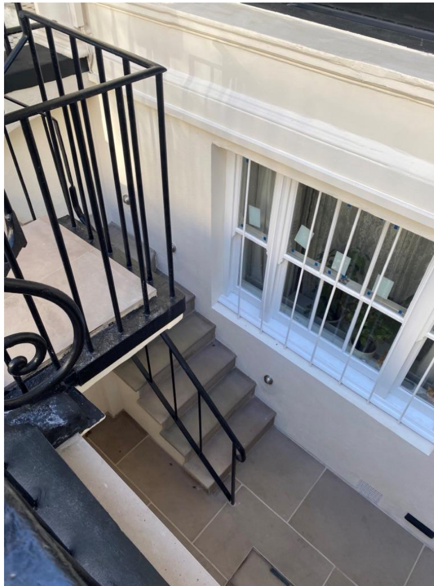
Reclad Supported LG Steps with safety lighting [after]
