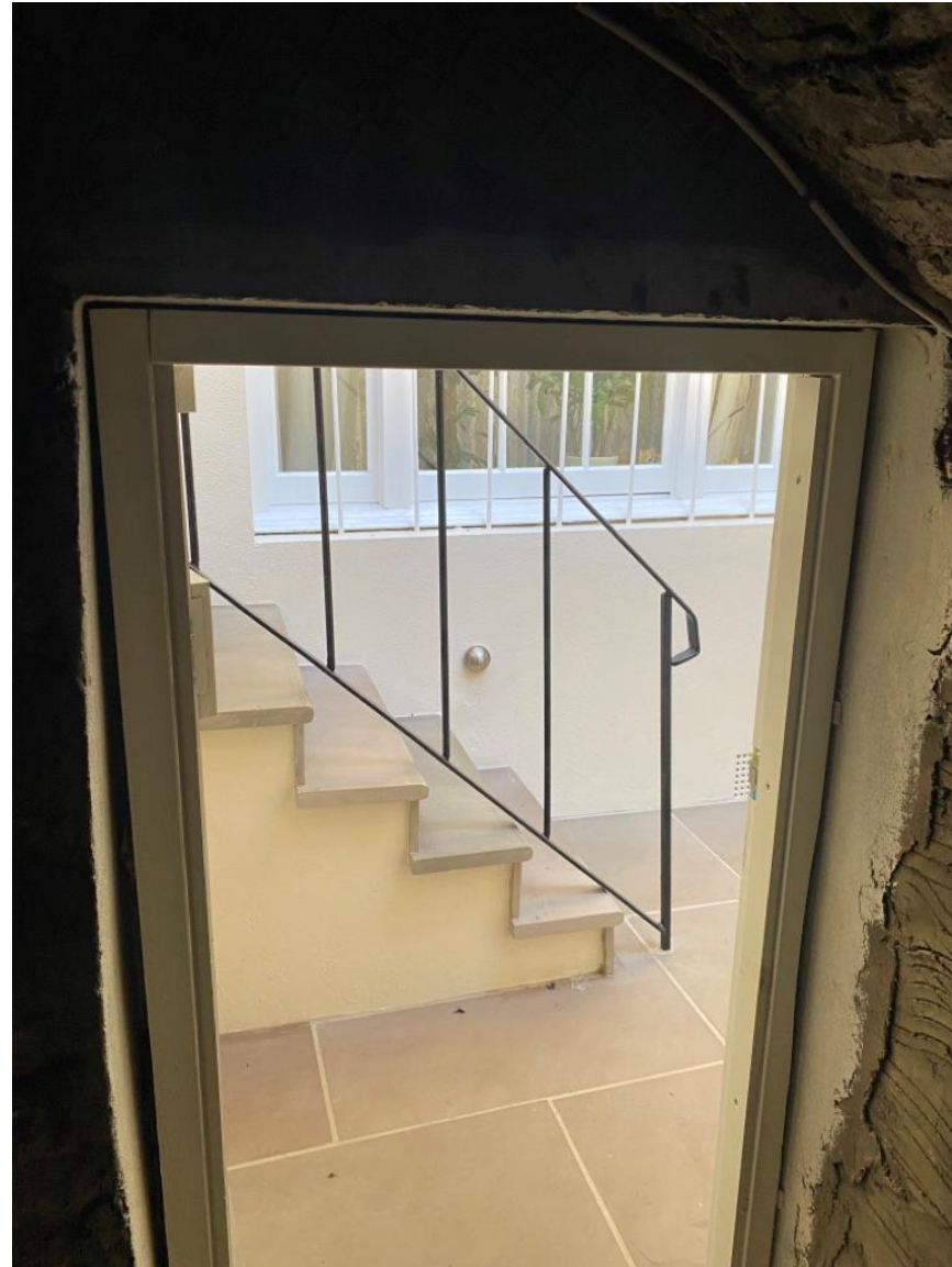
New Vault Lintels Internal [after]
