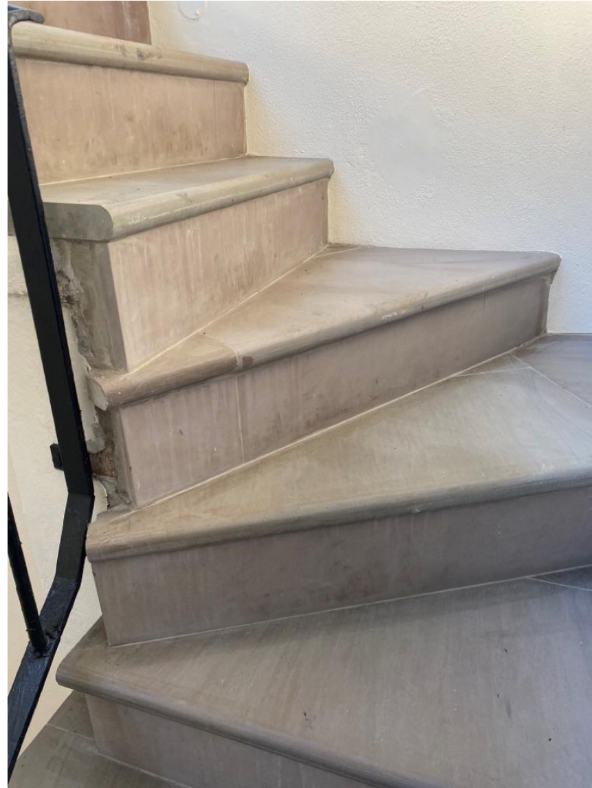
Structurally Supported Reclad Steps [after]
