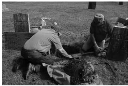
Del Gilpatrick & Bruce Nason fixing a sunken gravestone
