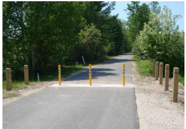
Figure 8 – An example of bollards used to restrict unauthorized access to the trail. Bright paint and reflective tape ensure that the bollards are visible to trail users.
