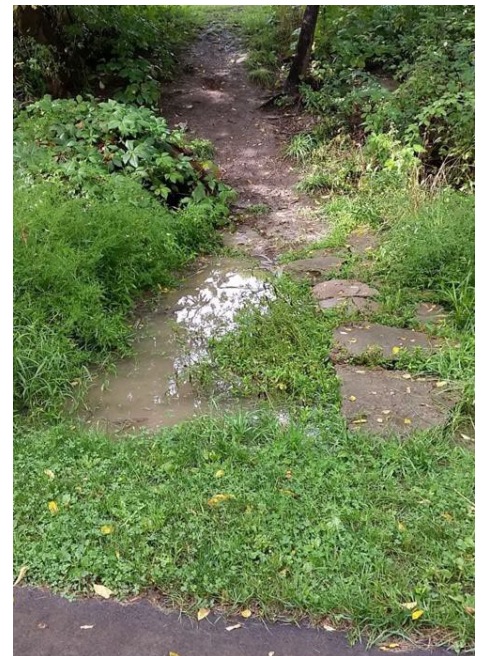
Figure 4 – Pavers placed by adjacent landowner to access the trail causing an interruption of proper drainage
