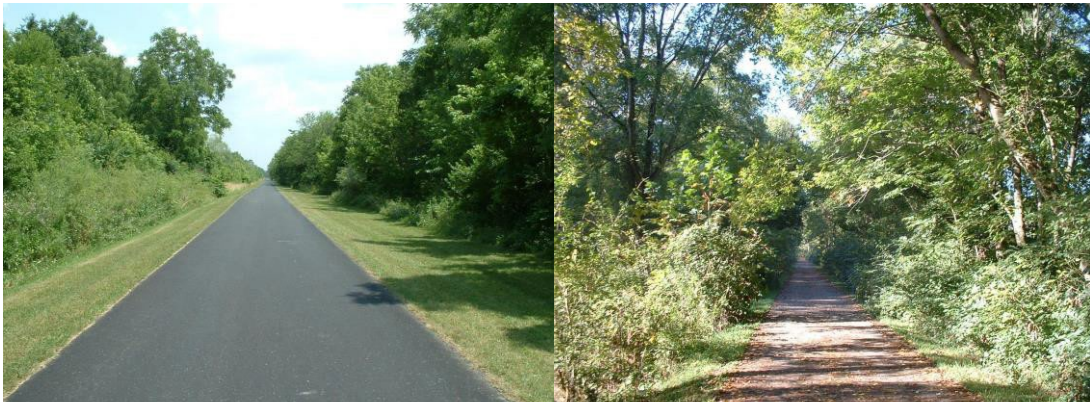
Figure 5 – A well maintained corridor, brushed and mowed, will protect the trail from roots and requires less major cutting of vegetation
