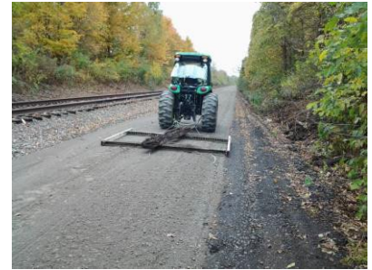
Figure 3 – Dragging an aggregate trail will smooth out holes and ruts and redistribute surface material.
