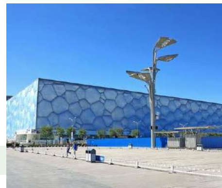
Water Cube (National Aquatics Center)
