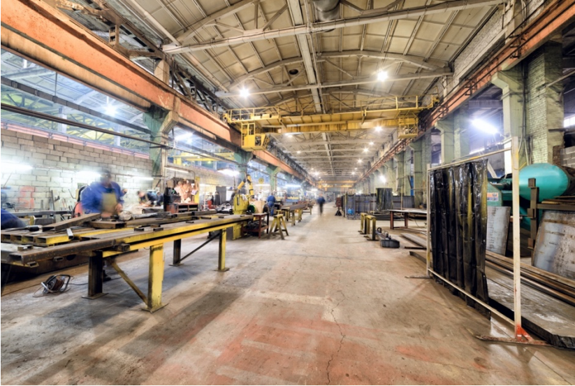
Figure 1: A Heavy Industrial Building
