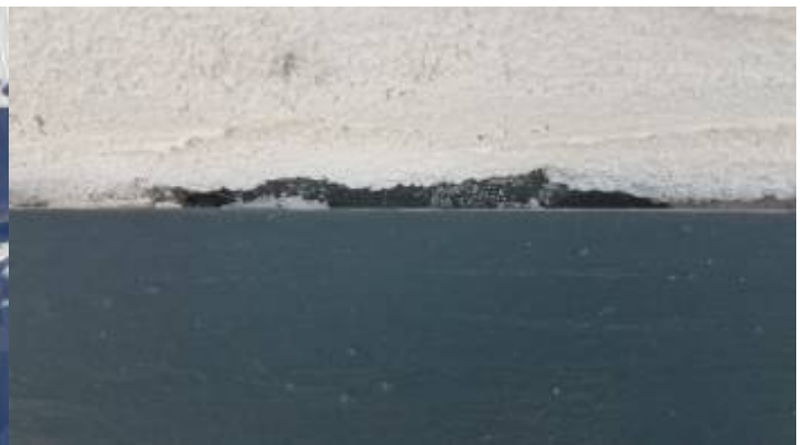
Exposed framing behind stucco. No flashing seen between balcony and stucco
