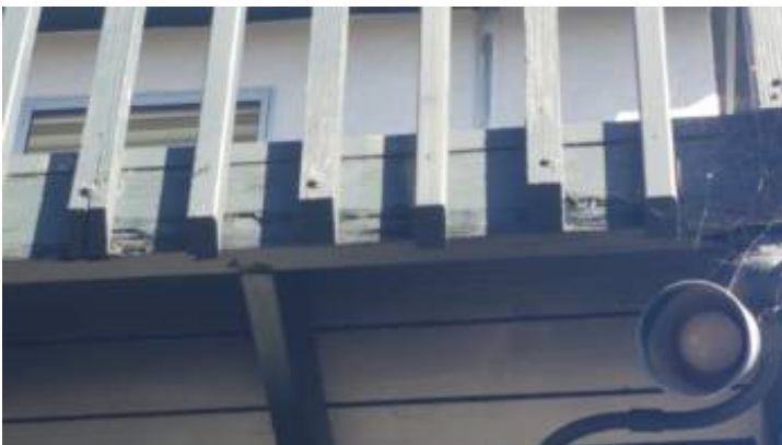
weathered wood surface at balcony framing
