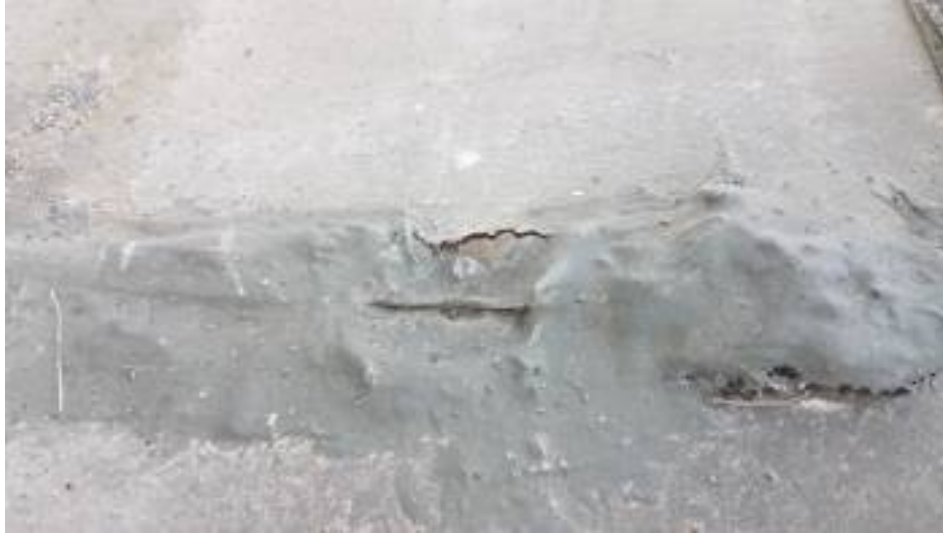
damaged seam at valley flashing
