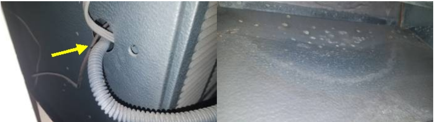
Fuel line susceptible to damage
