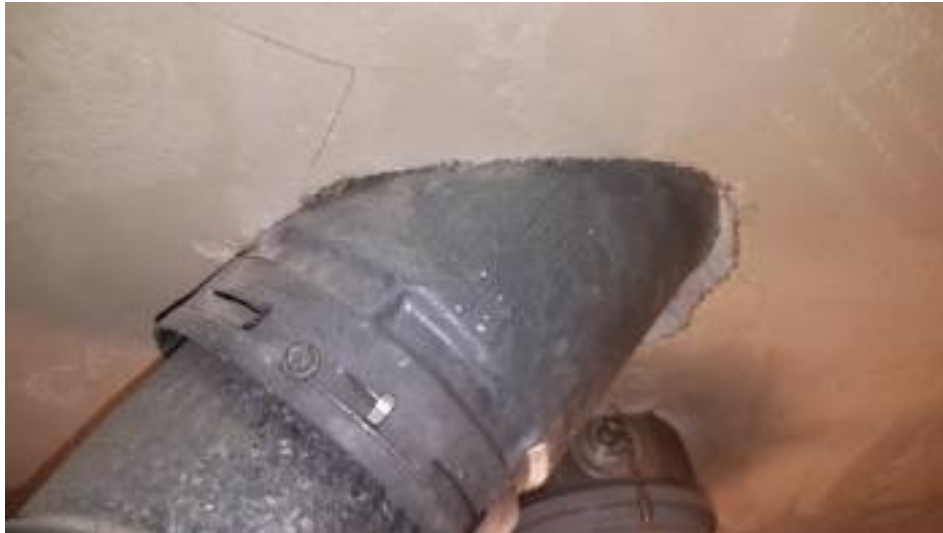
improper clearance to combustibles
