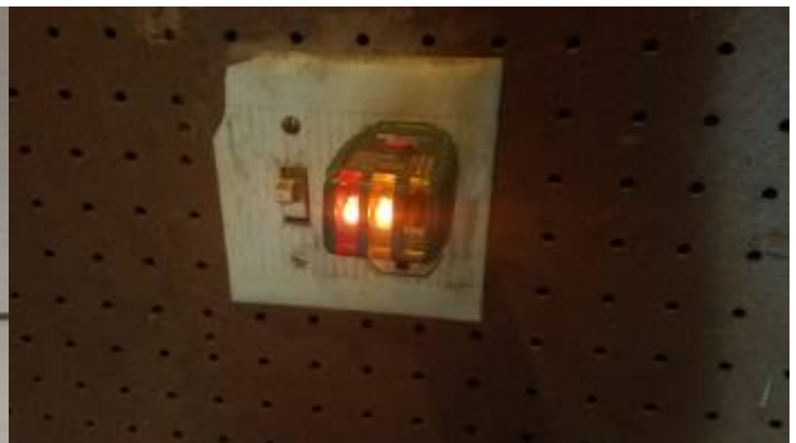
Receptacle with reverse polarity in garage
