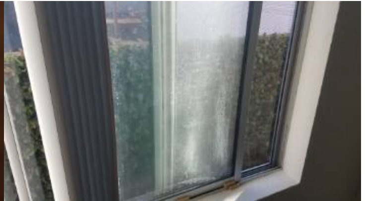
failed seal at master bedroom window
