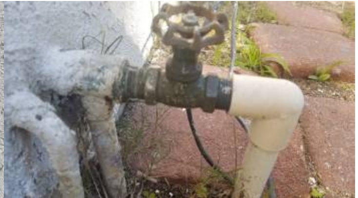
Leaking shut off valve
