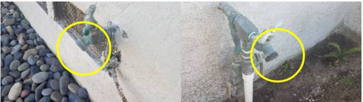
Missing Anti-Siphon Valve
