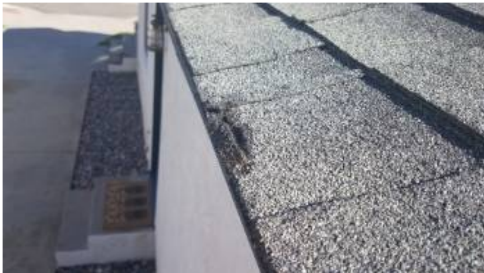
damaged shingle
