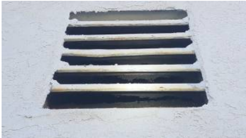
Vent screen damaged
