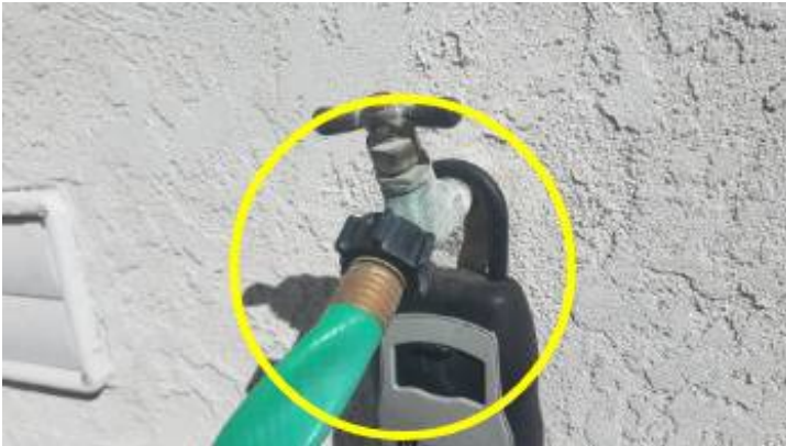
Missing Anti-Siphon Valve
