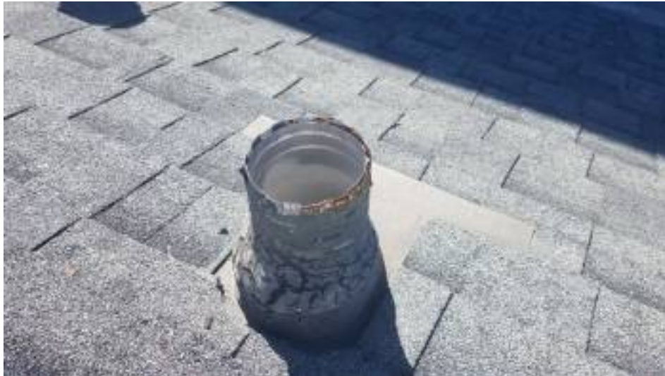
rain cap missing on furnace exhaust vent
