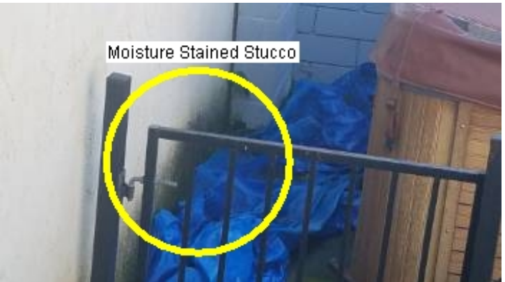
Moisture Stained Stucco exterior wall corresponding with moisture entry in garage
