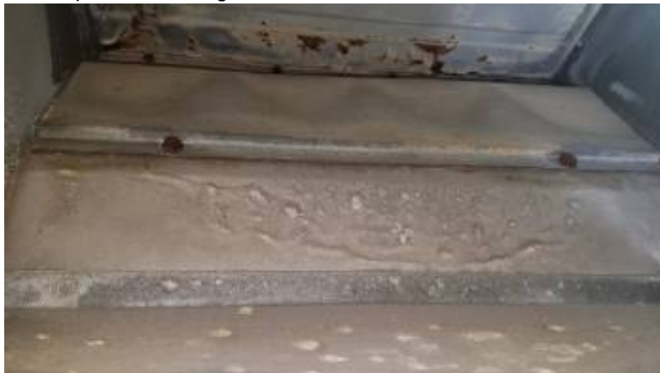
rust seen inside furnace cabinet
