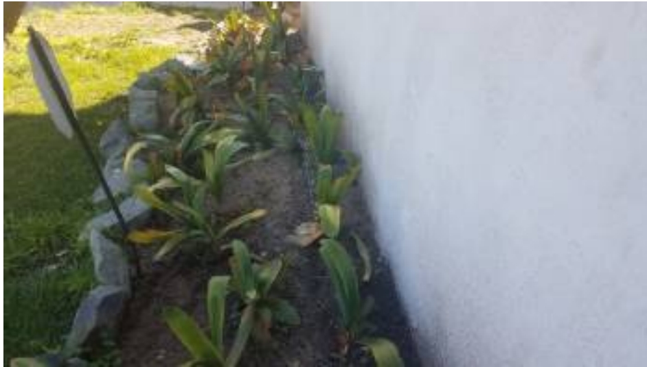
Poor grading at foundation
