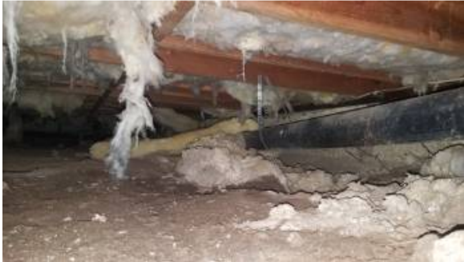
Insulation detached from floor in crawlspace
