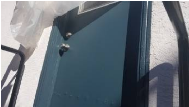
Moisture damage at staples
