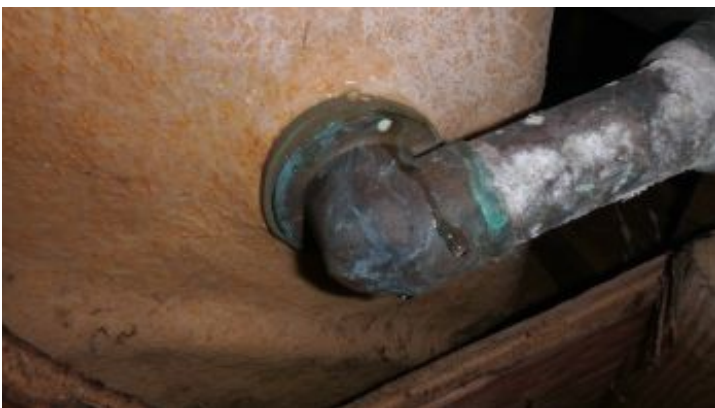
Leak was seen at master bathroom tub drain
