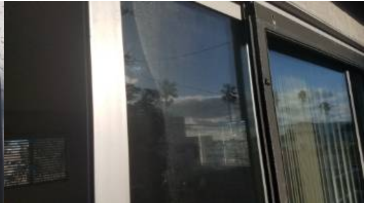
bad seal in upstairs sliding glass dual pane door
