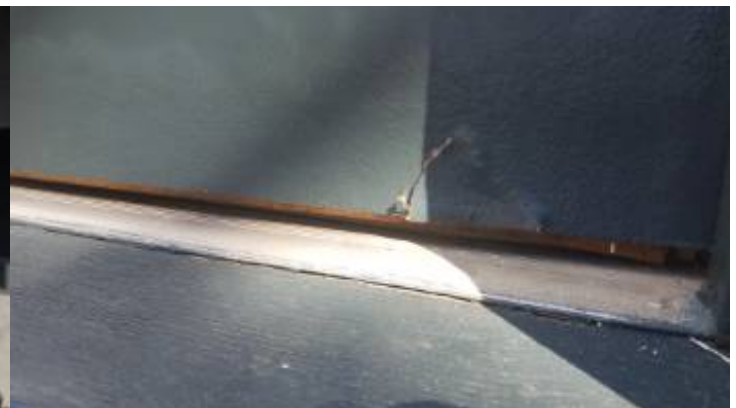
moisture damage at bottom of door
