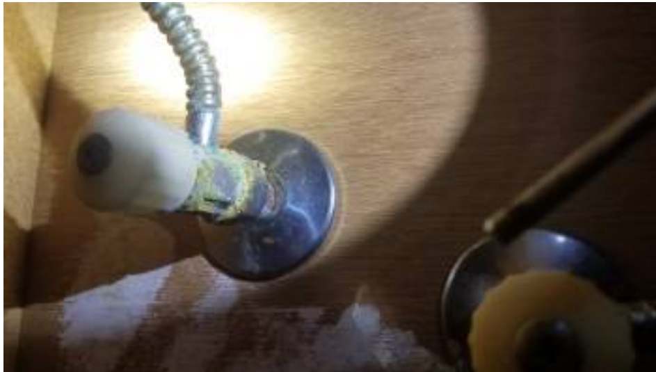
corrosion at master bathroom sink shut off valve
