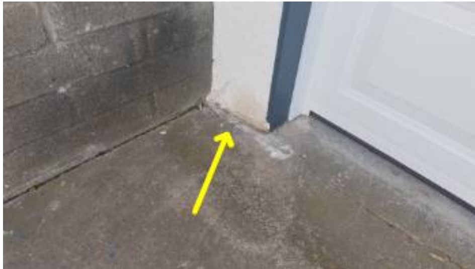
Improper slope
