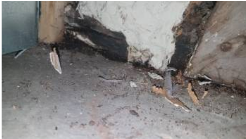
Moisture intrusion at garage sill plate next to door
