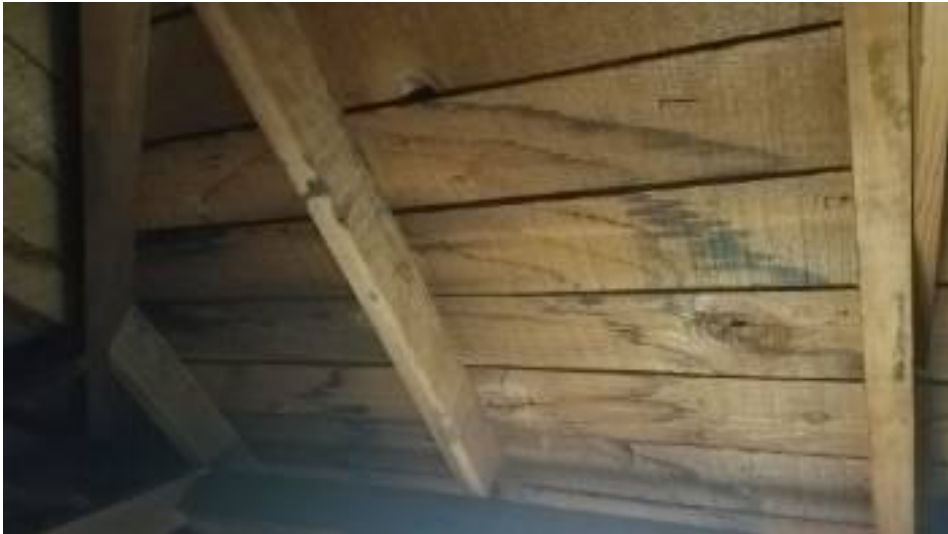
Staining seen on roof decking in attic
