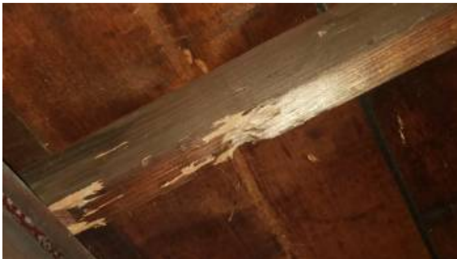
damaged joist in garage
