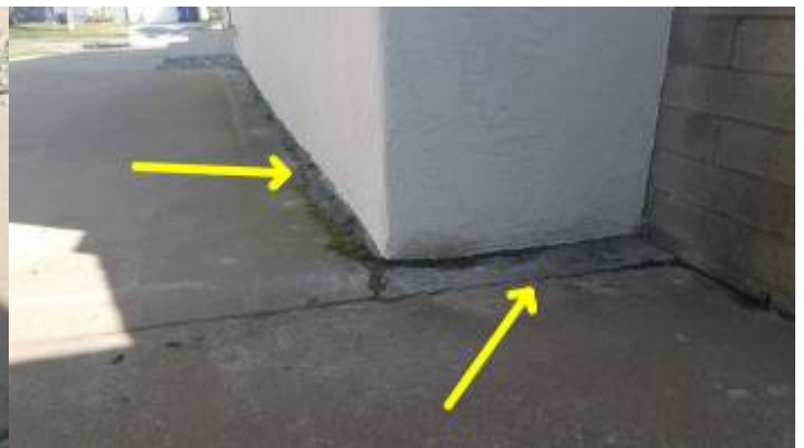
improper slope
