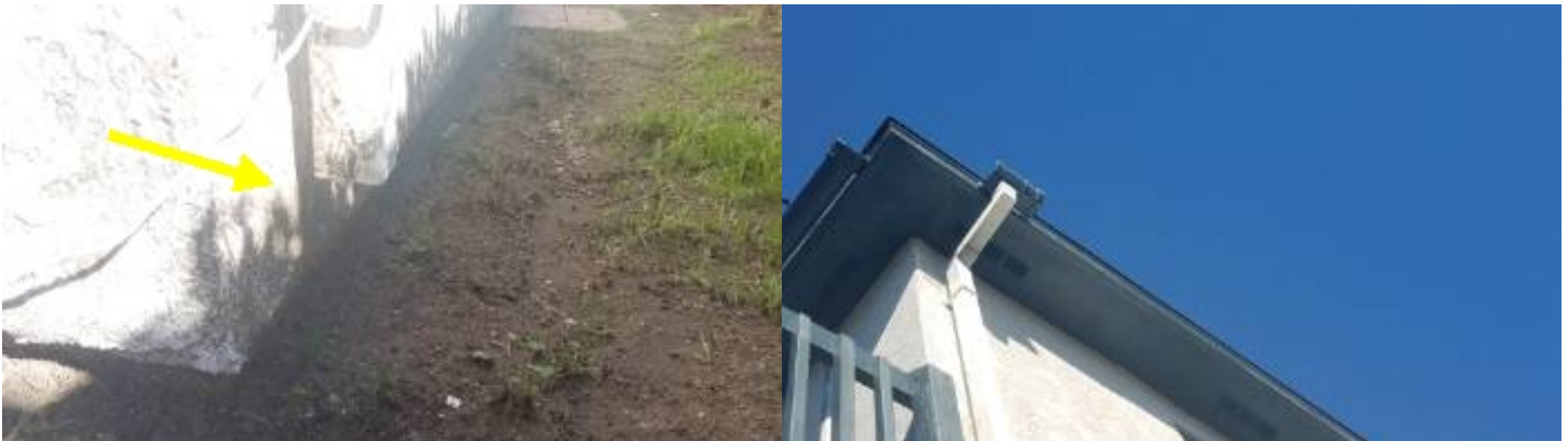
Downspout Next To Foundation
