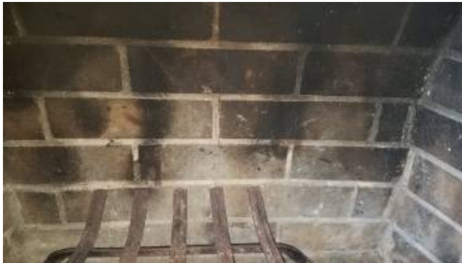
Crack in firebrick
