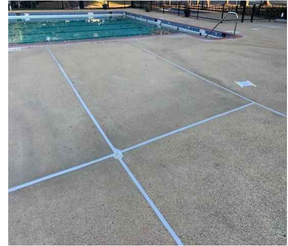
Replaced expansion joints
