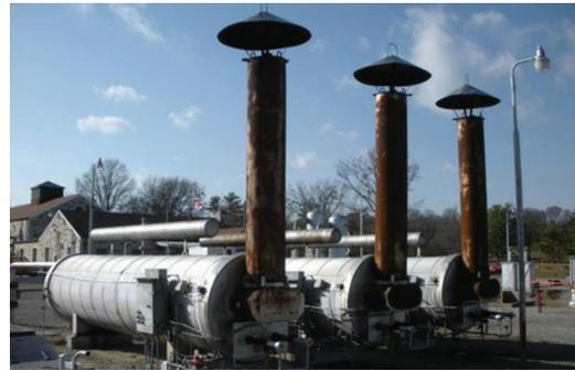
Example water bath line heater installation
