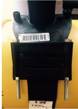
Correct clamping of belt strap
