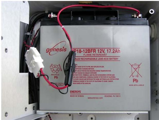
If the battery voltage is between 11.5 and 12.0 volts, the SunSaver will sometimes power-up during initial installation in the LVD state. This will automatically clear when the battery voltage rises above 12.6volts. If the battery voltage is above 11.5V the LVD can be reset
