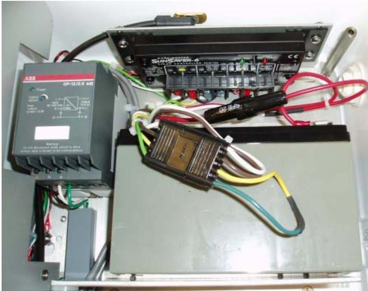
Figure 28 Battery, Connector, and Fuse
