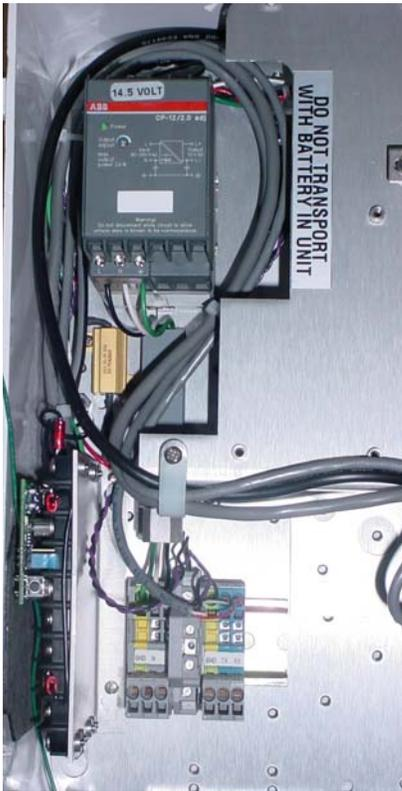
The AC Hybrid power source includes a 12VDC adjustable power supply, 7AH rechargeable sealed lead acid backup battery, and SunSaver Solar Controller. The power supply will look similar but may not be identical than the one in Figure 24: AC Power. The 12VDC power supply is adjusted to 14.5VDC to provide optimum power to the SunSaver Solar controller to charge the battery. The SunSaver Solar Controller and battery are located behind the pivot panel.
