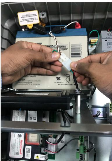
4. Close the battery mount bracket flip cover by quarter turning the screw.
