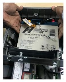
4. Close the battery mount bracket flip cover by quarter turning the screw.
