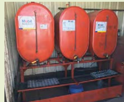
Metal containment for drums/tanks
