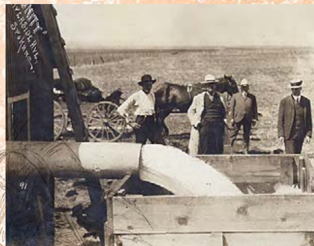
Modern Irrigation & Land Co. 3,000 gpm, 1908.
