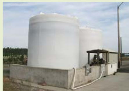
Concrete containment
