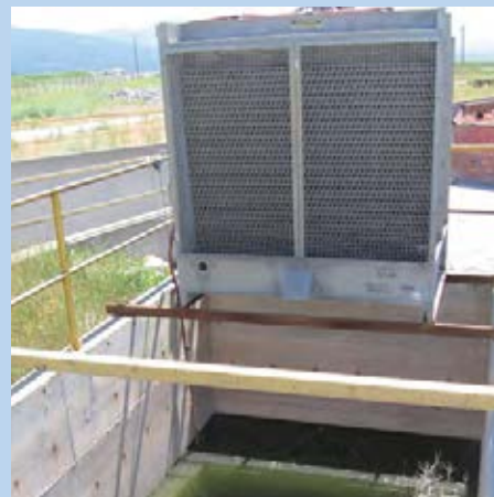
Approved wastewater retention pit with mechanical evaporator
