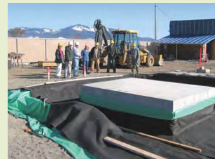
Poly-geotextile containment
