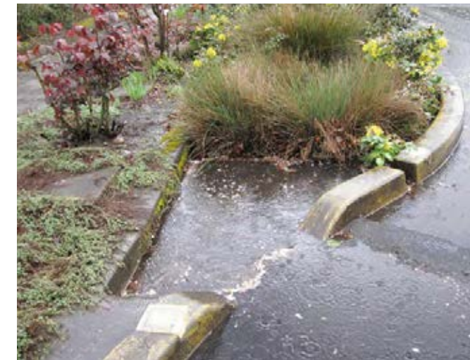
Bioretention facility in Spokane
