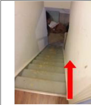
Missing handrail. Recommend installing one for safety.
