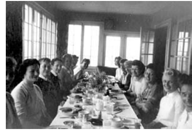
Interior of Building Addition #1, a sixty-foot-long dining area.
