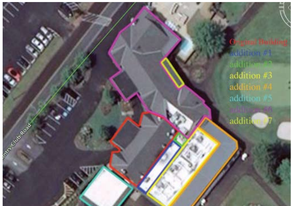
Modern aerial view of facility envelope. The various additions are outlined in separate colors as indexed right.
