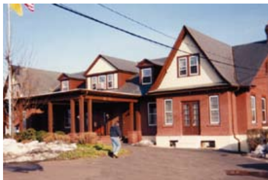
The clubhouse original facade remains basically unchanged. The double doors shown above were "bricked in" and three middle dormers were removed in 1994.
