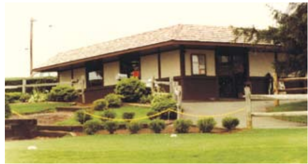
Building Addition #5—Pro Shop.
