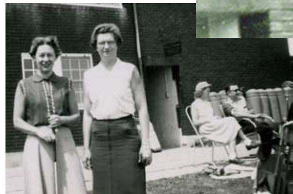
Building Addition #2. The Golf Shop Entrance is shown in the background. Note the sign above the entrance that says “Golf Shop, Jack Robinson, Professional.” (1954)
