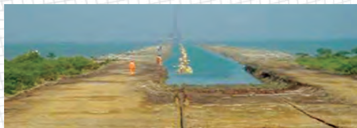
Installation of oil pipeline in the Middle East using Salvage Pontoons 6,000 lbs.
