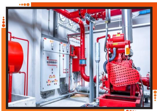
We are engaged in wide range of Automatic Fire Hydrant Systems which is designed with high quality components. The landing valves & fire hose cabinets are provided for the use of occupants to fight small fires. Water flowing through the sprinkler orifice strikes the sprinkler deflector, forming a uniform spray pattern to extinguish or control the fire
