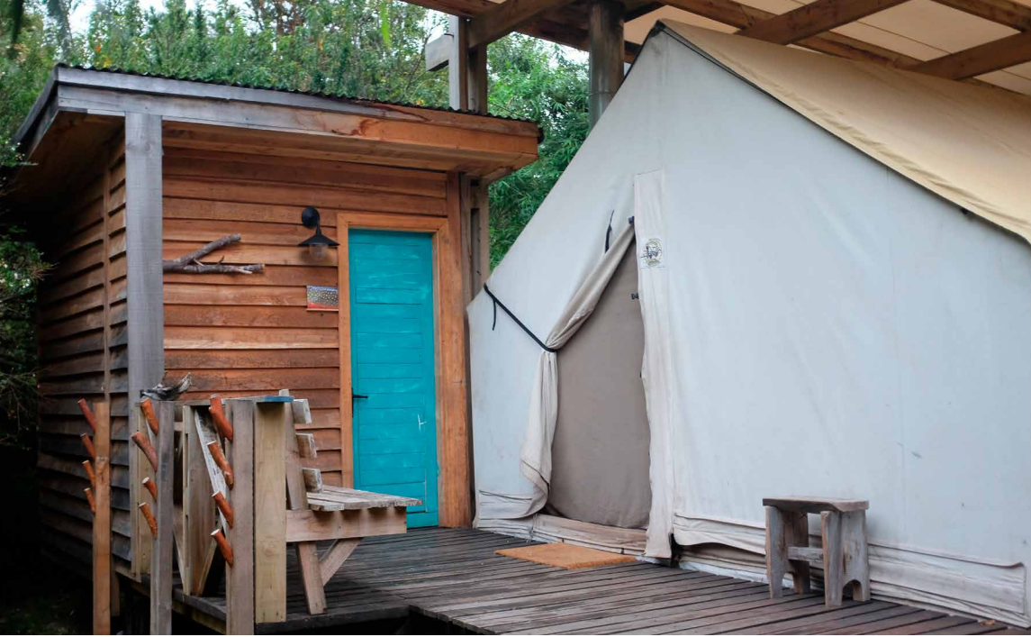
Left: one of the semi-permanent glamping wall tents with attached restroom and rigging area
