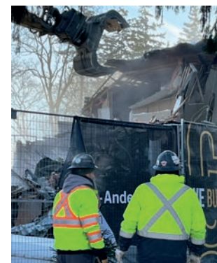
Workers watch as an excavator takes initial bites out of a heritage home on Victoria Street, demolished as part of the Shaw's real estate expansion.
