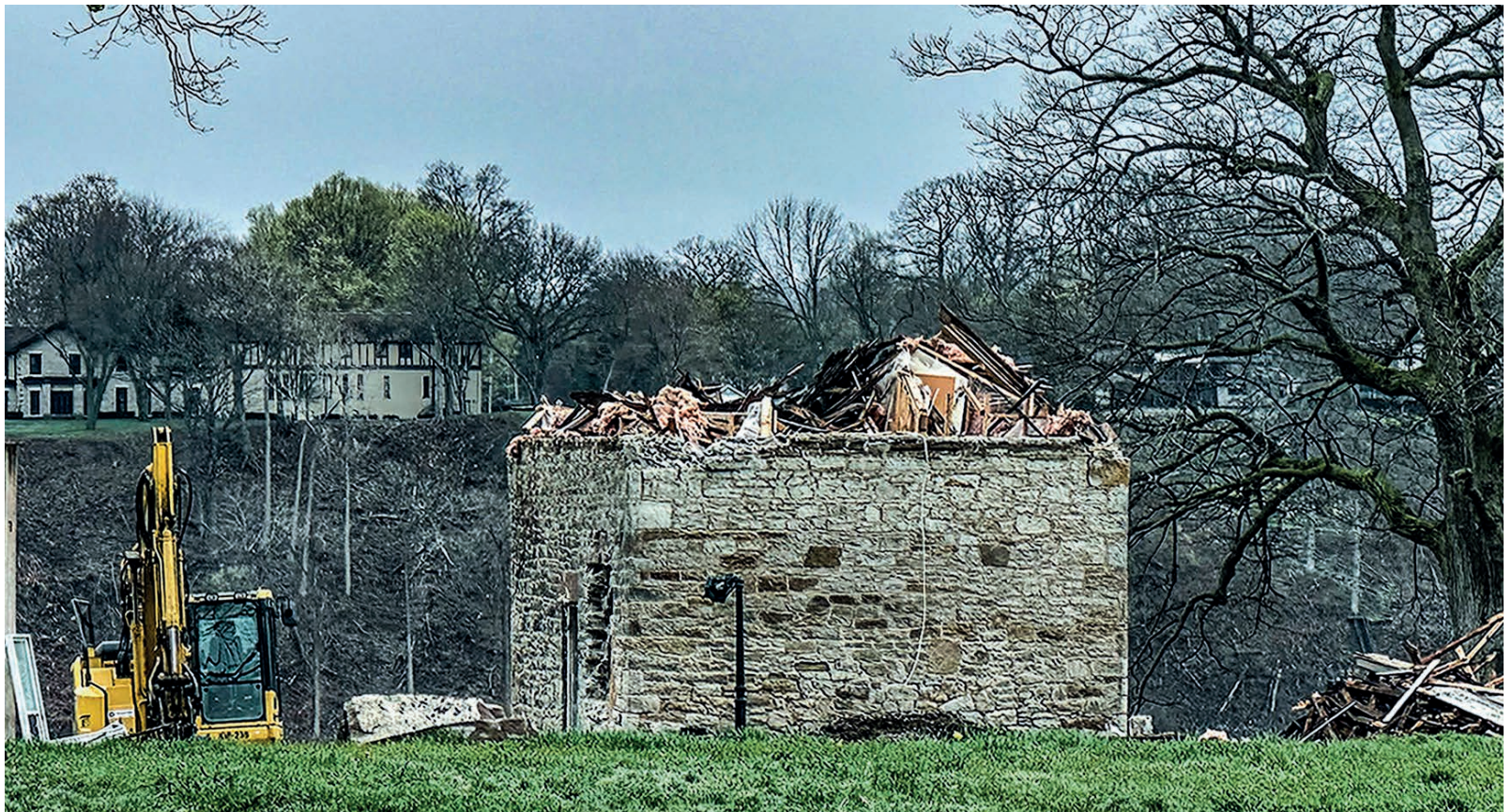
The Town of Niagara-on-the-Lake issued a stop-work order on a stone structure located on 14785 Niagara River Pkwy. after a complaint about activity on the property. The work to demolish the roof of the building had started without required permits or approvals. BRIAN MARSHALL
