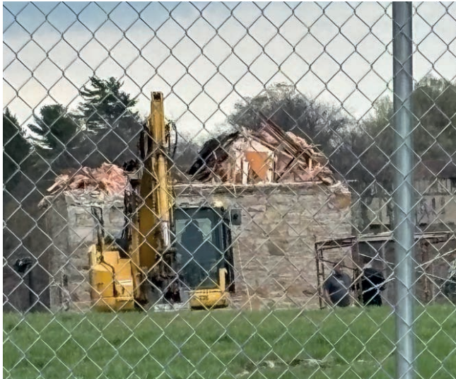
No one who understands construction would use a backhoe to remove a roof unless the end game was to demolish the existing building, writes Brian Marshall.
