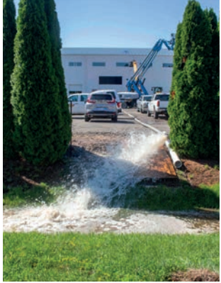
Water being pumped out onto East & West Line. FILE
